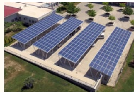
In 2022, with the electricity tariff change 1.66%; i.e. 860,269.72 TL savings per year.
