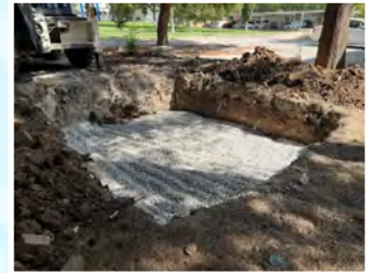
Construction of rain water pool
