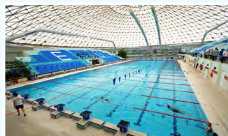
Treatment of Olympic-sized swimming pool
