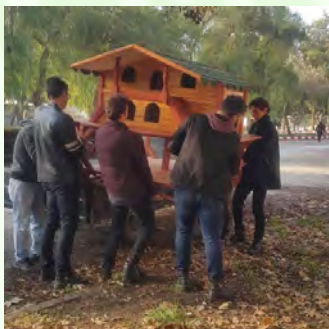
Construction of shelters
