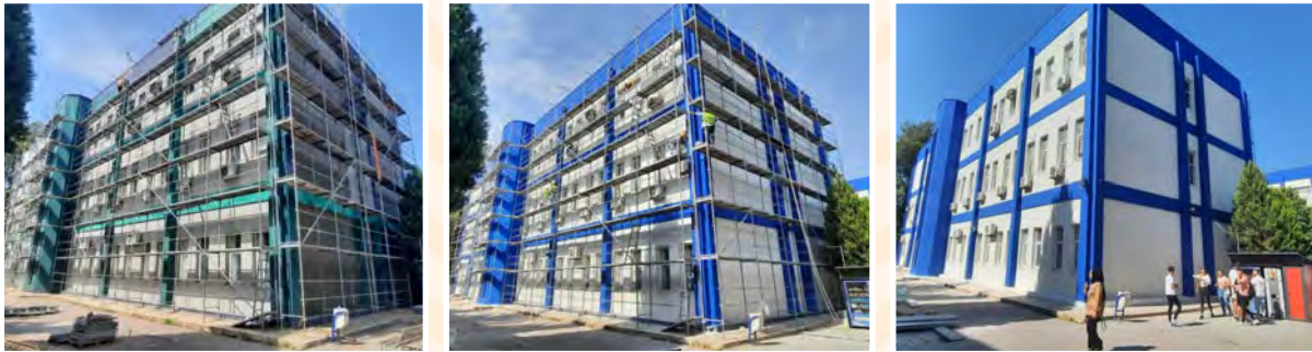
Facade restoration of Ege Vocational School
