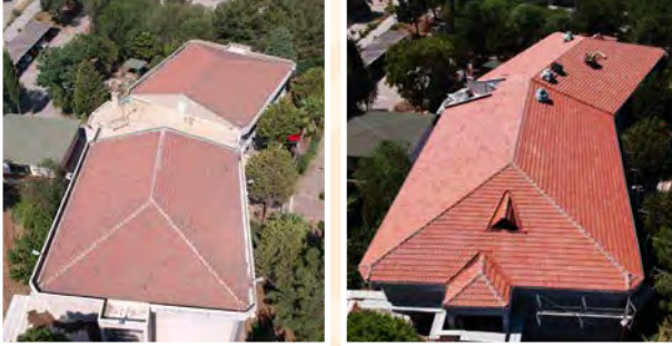
Roof reconstruction of Emel Akın Vocational School
